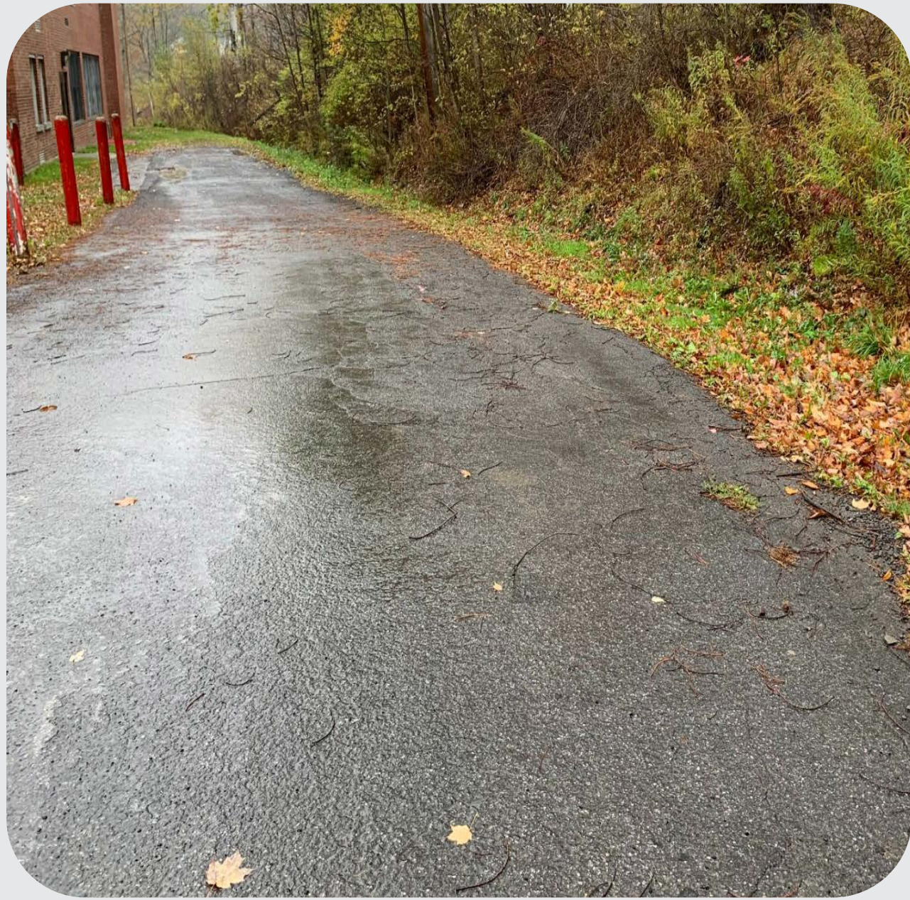
Excess Surface Water at Swale
