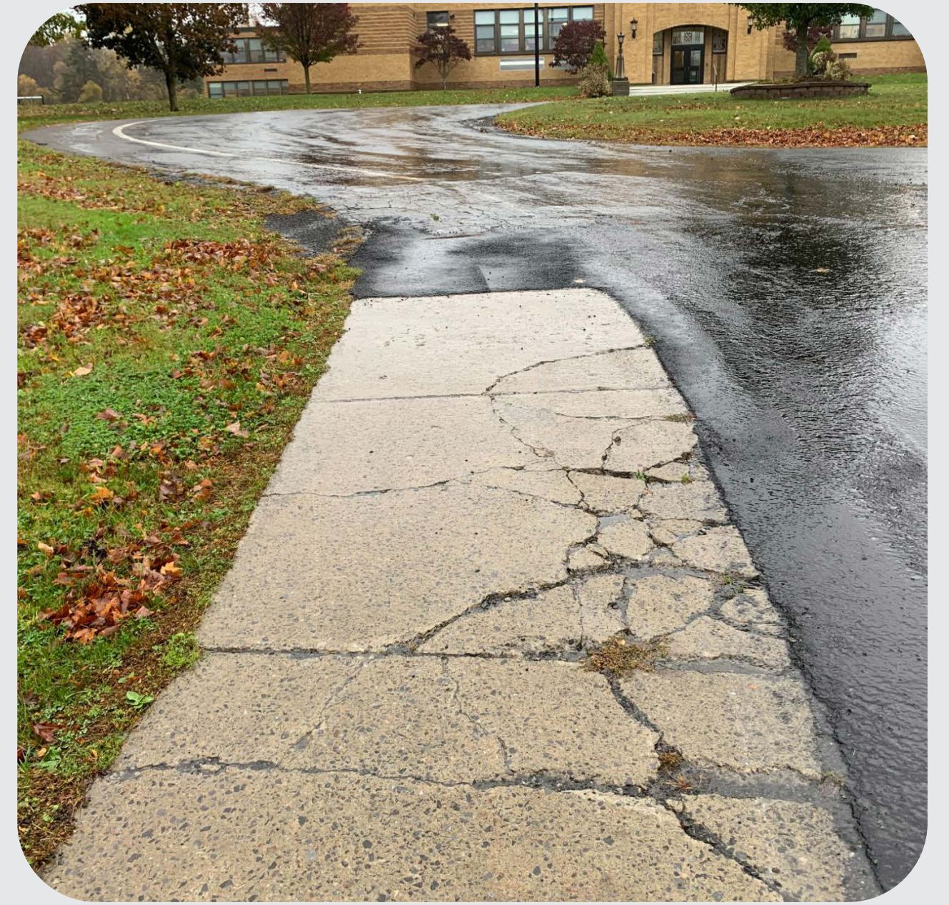
Unsafe Sidewalk Conditions
