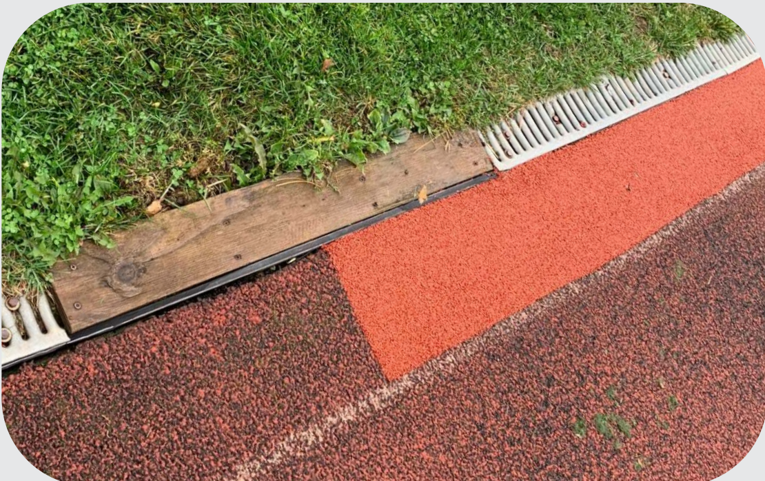
Failing Track Drainage
